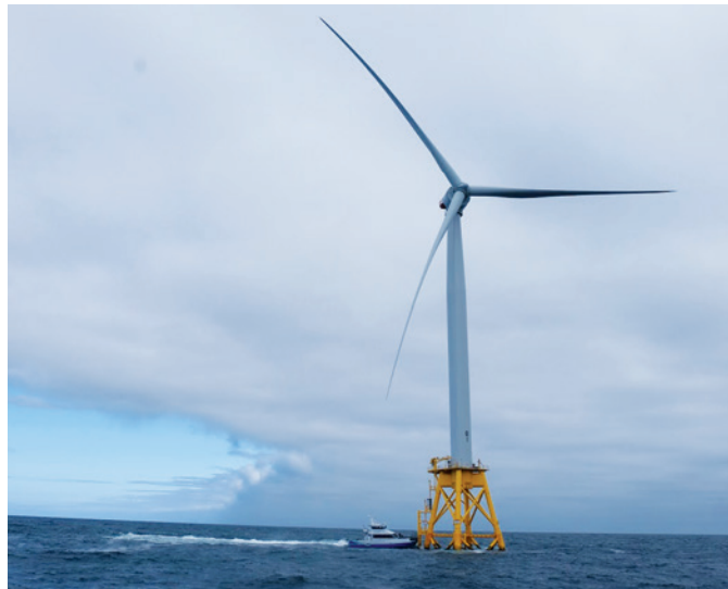
Block Island Tour (Rhode Island)–First USA offshore wind farm. Photo credit: WDI
